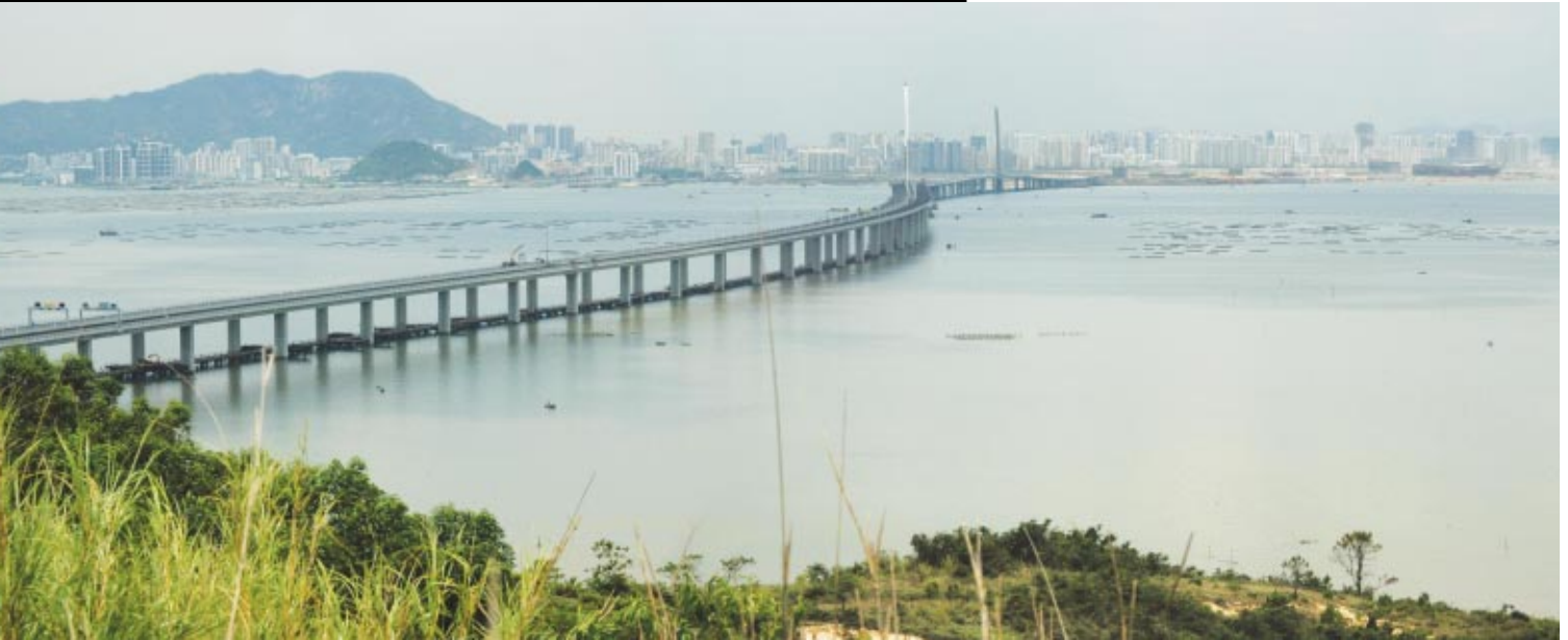
Viaduct and bridge structure basically completed as seen in late 2006. The temporary access bridge on the underside of the viaduct would soon be dismantled
