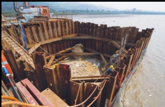
Close up view of a sheet-pile cofferdam at its formation level. The pile heads were exposed ready for the forming of the pile cap for the portal pier
