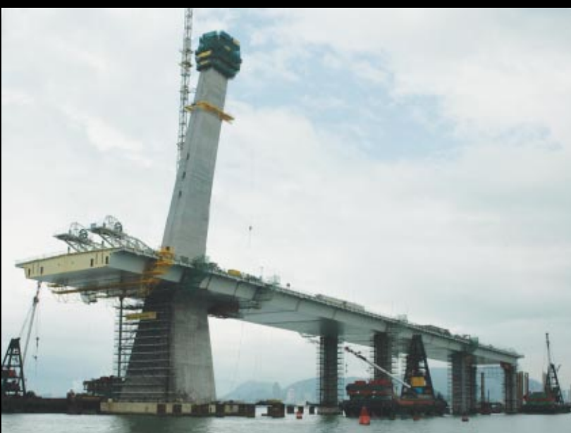
The construction of the cable-stay bridge and the back span as seen in July 2005. The 158 m tower was still under construction at the same time meeting with the progress of the installation of the main span. The bridge has a main span of 210 m and a back span of 99 m. There are also two 74.5 m spans that are proceeding and structurally continuous with the back span. The photo shows only the back span and the two continuous spans already lifted onto the deck level and supported by piers at the early stage pending for the installation and stressing of the stay cables
