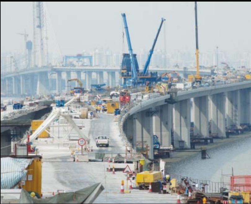
After serving for almost 15 months, the launching gantry was dismantled and removed upon the final completion of the viaduct as seen in September 2006
