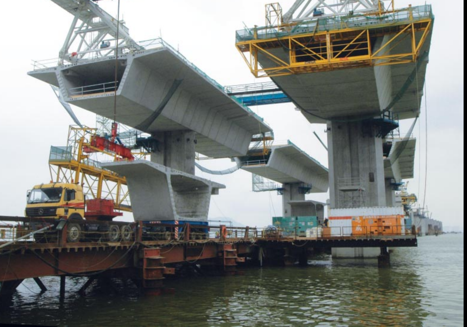
The use of simple gantry frame to construct the viaduct using balanced-cantilever method was adopted for section within the reach of the TAB. Precast segment weighting more than 50 tons each can be transported conveniently by lorry trailer using the temporary roadway. The arrangement has the benefit to save time for this can allow the carrying out of work at multi-locations, as well as to save cost using simpler and cheaper equipments
