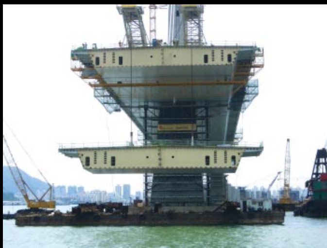
Lifting of a segment of the main span from barge
