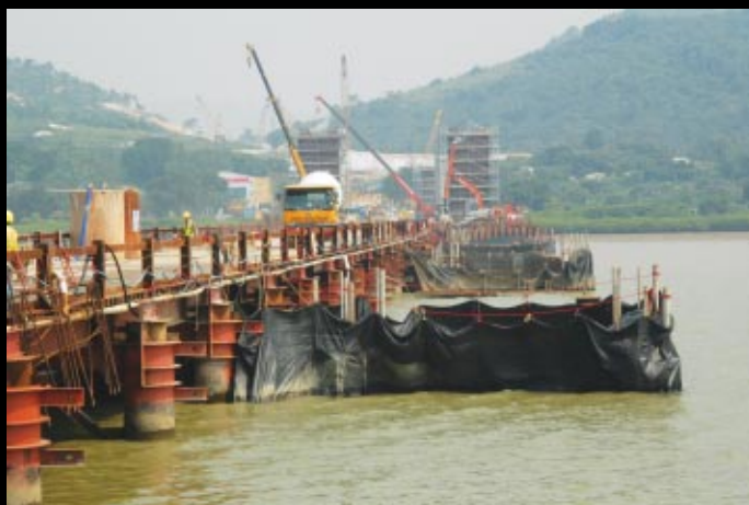
Viewing towards Ngau Hom Shek (鰲磡石) from one of the work station with the supporting temporary steel piles on the underside of the access roadway clearly seen. Since Deep Bay is environmentally sensitive, silt-screen was erected (photo centre) during the bore-pile forming process in order to avoid the pollution of the seawater by silt and mud
