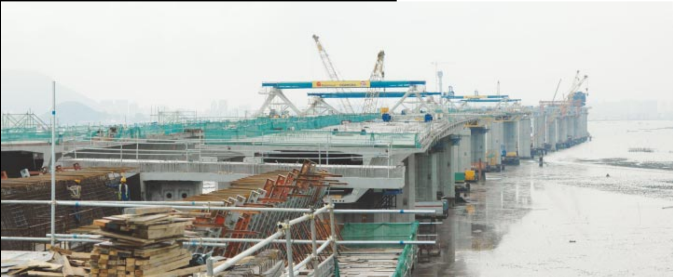
Panoramic view on the deck level of the viaduct during the low tidal period near the landside at Ngau Hom Shek. The semi-marshland condition of the nearby environment can be seen on the right
