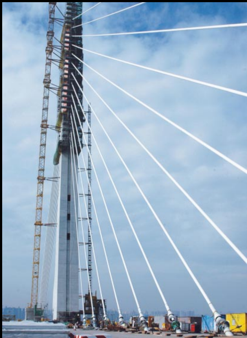
View of the bridge tower with the stay-cable for supporting the deck of the main-span in place and temporary stressed. There are 13 pairs of stay cables arranged under a single-plane configuration. The cables are used to balance the large moments caused by the main span onto the inclined bridge tower and the back span
