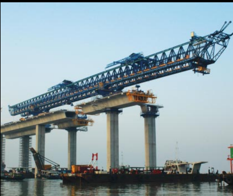
Launching gantry as viewed from sea-level under its operating condition. Note the team of servicing support formed by barges and other work boats stationed around the gantry to assist in the viaduct installation
