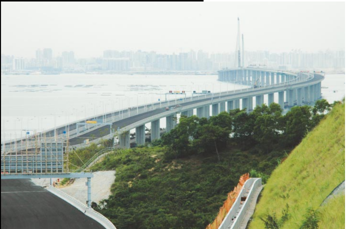
The 3.4 km long carriageway of Western Corridor on Hong Kong marine boundary as viewed from an upper ground in Ngau Hom Shek
