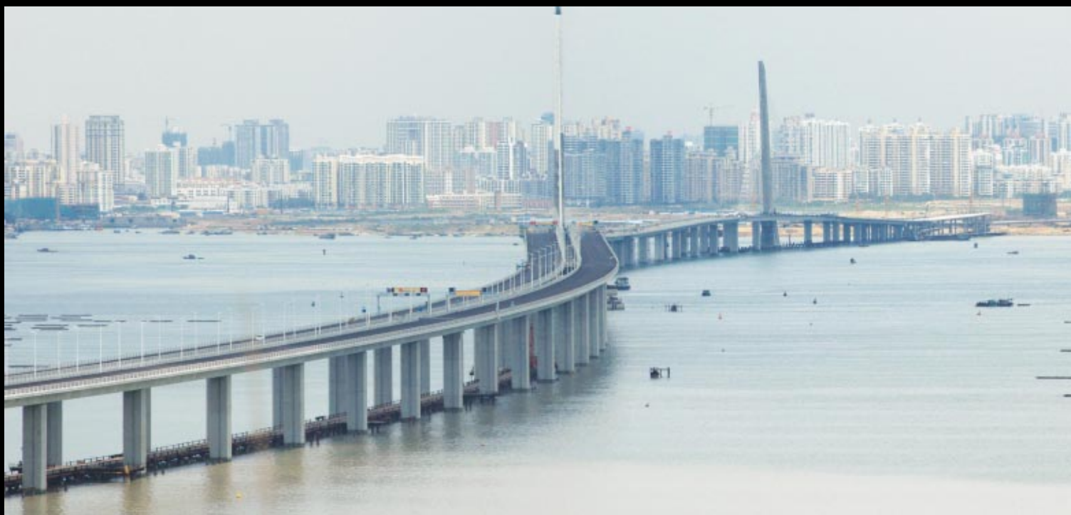
Close up look at the cable-stay bridges constructed by Hong Kong and China with Shekou of Shenzhen forming the background in the photo. The north and south navigation channel are situated under the main span of both bridges
