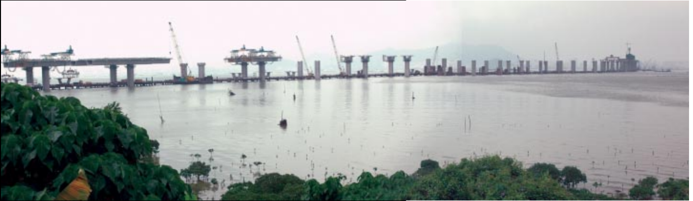
Viewing from the landside, the entire access roadway with most of the piers for the portal frames being completed. Part of the viaduct sections constructed with the help of launching gantries can be seen in various locations
