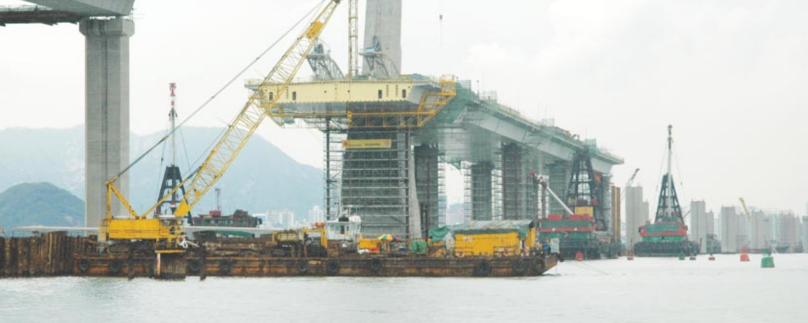
Side view of the back spans. The main span at the front of the bridge tower was still pending for the completion of the upper structure of the bridge tower where the anchor head for the stay-cable would be located
