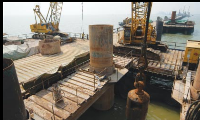
Close-up view of a work station where a portal frame situated. All the equipments can be seen in working position for the forming of a bore-pile cluster
