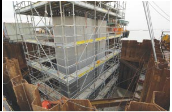
The first section of the portal pier ascending from the cap ready for the placing of the formwork for the onward pier section
