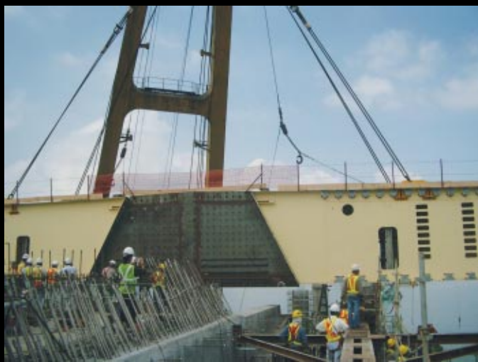
Placing the first segment onto the deck level of bridge tower. The coupling bars anchored in the tower structure and the shear studs on the sides of the segment would embed the deck segment rigidly and in one-piece at a later stage
