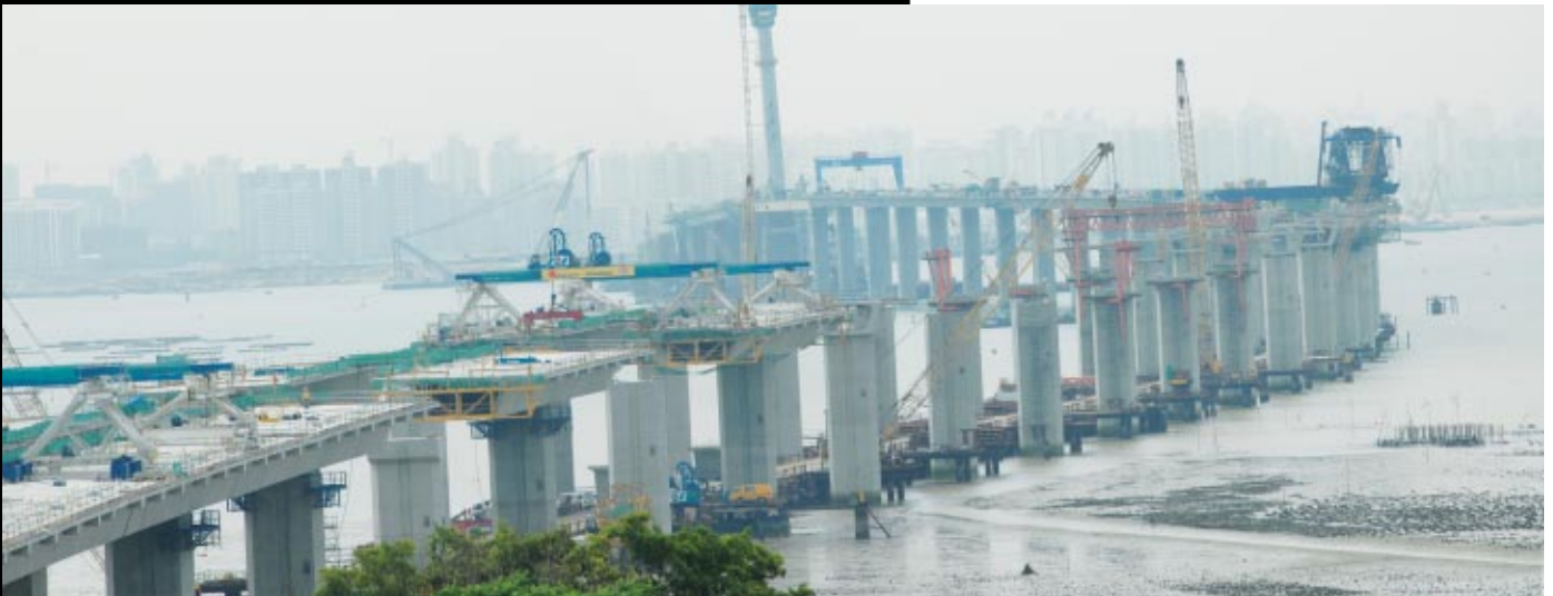
Overview of the viaduct construction at its peak period in late 2005. At that moment, there were more than 6 sets of launching machines in various size and capacity under operation, including the 175 m long launching gantry working mainly outside the temporary access bridge
