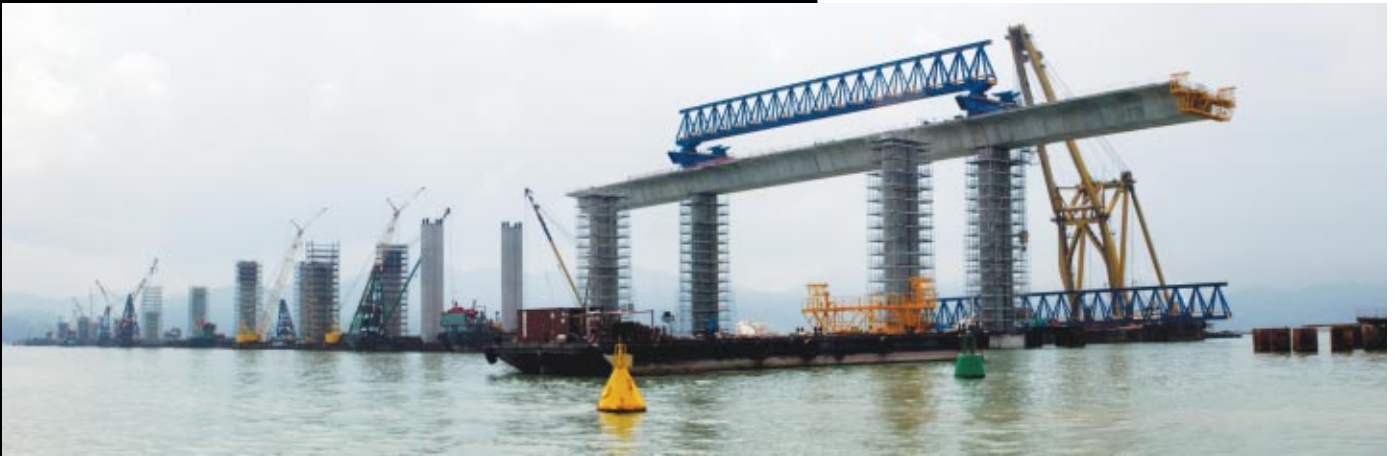
The erection of the first set of launching gantry as seen in October 2004. The first span of viaduct formed in advance by balanced-cantilever method, was used as the work station to support the installation of the gantry
