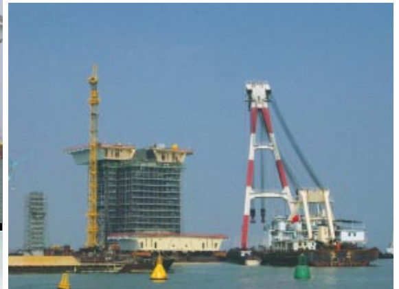
The lower portion of main tower of the bridge with the first deck segment placed in position. The tower structure would continue upward working at the same time with the back span, which was prefabricated and lifted to the deck level in one section and field weld afterward
