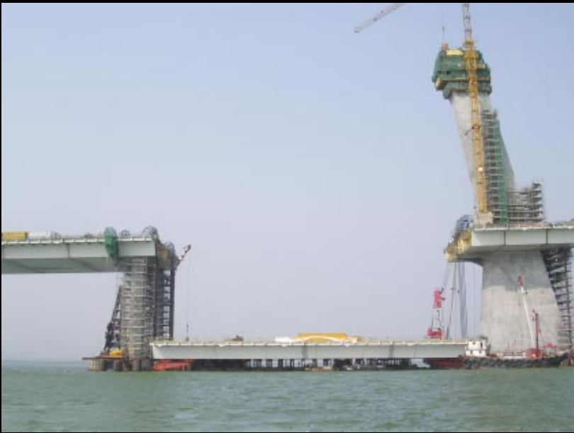
The prefabricated back span deck section mounted onto 4 sets of strand jack ready for lifting to the deck level
