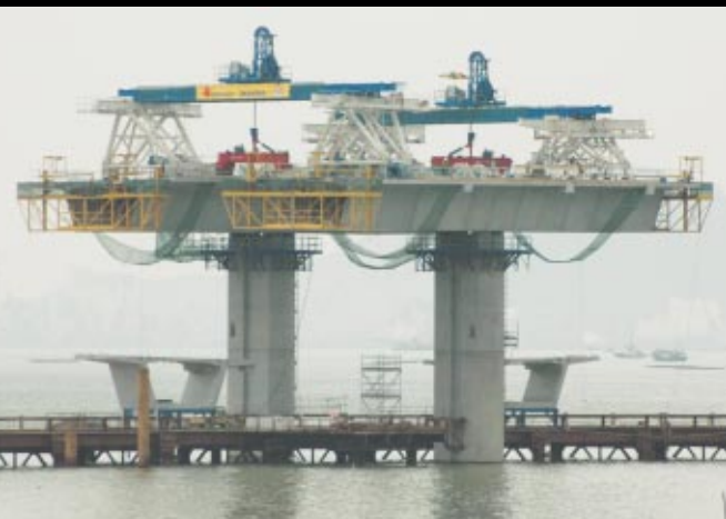
The gantry frame as viewed from the side. A set of strand jack was equipped at top of the gantry frame for the lifting of precast segment. Rollers and sliding tracks are provided in the gantry system for the concise positioning of the segment during installation
