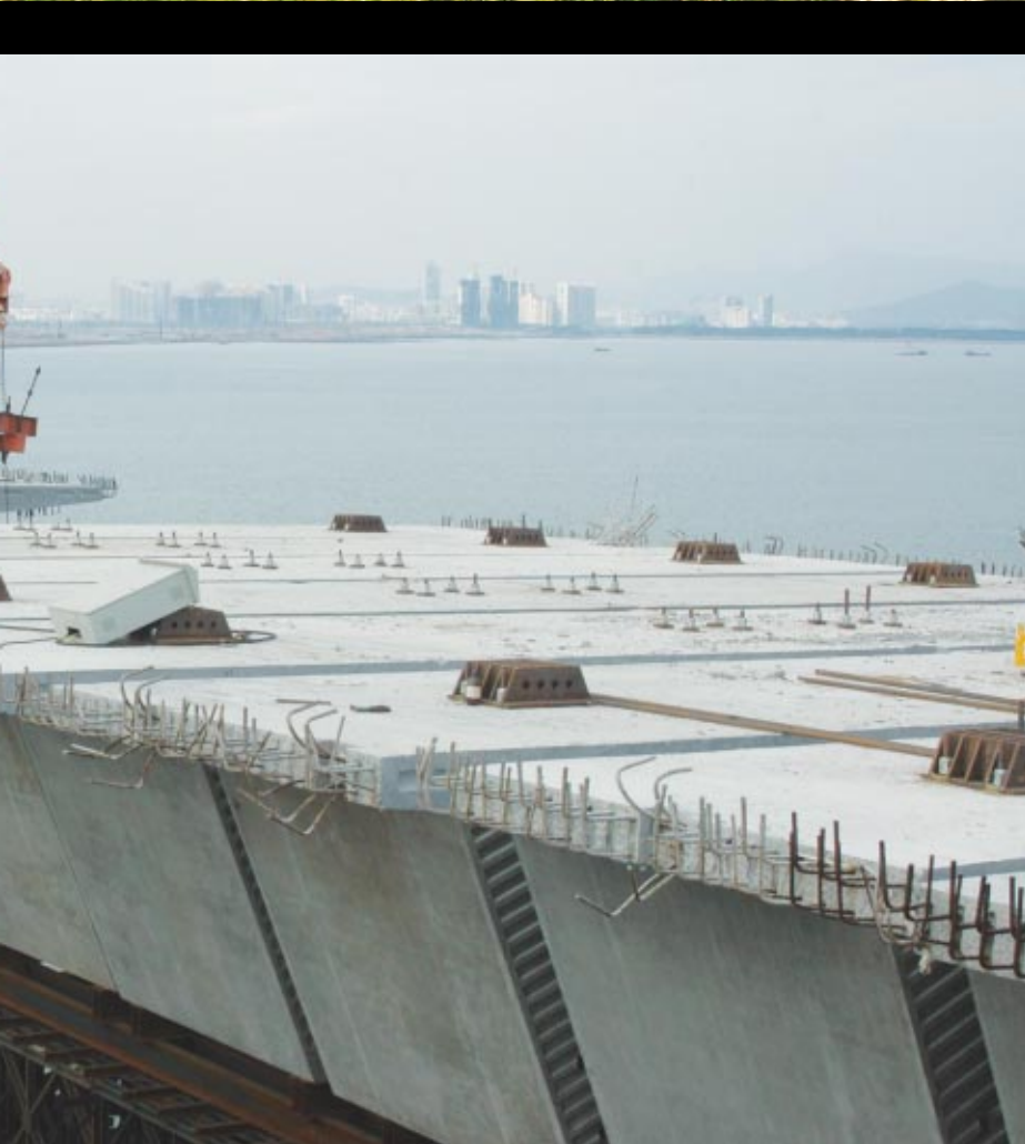
Close up on the segment installation detail under the practice on China side. Similar lifting frame was also employed at the same time with the in-situ installation with precast segment placed onto falsework (temporary platform) for final connecting onto pier heads (photo right)
