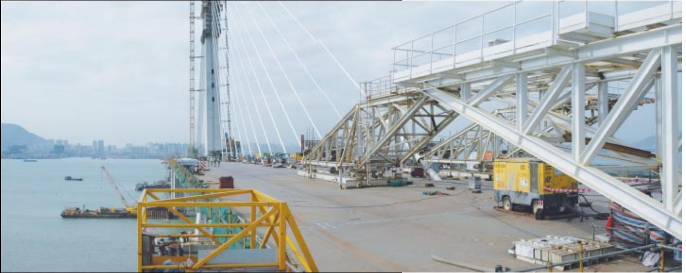
View on the deck of main span with a heavy-lift gantry positioned and anchored for the onward lifting of the next prefabricated deck segment
