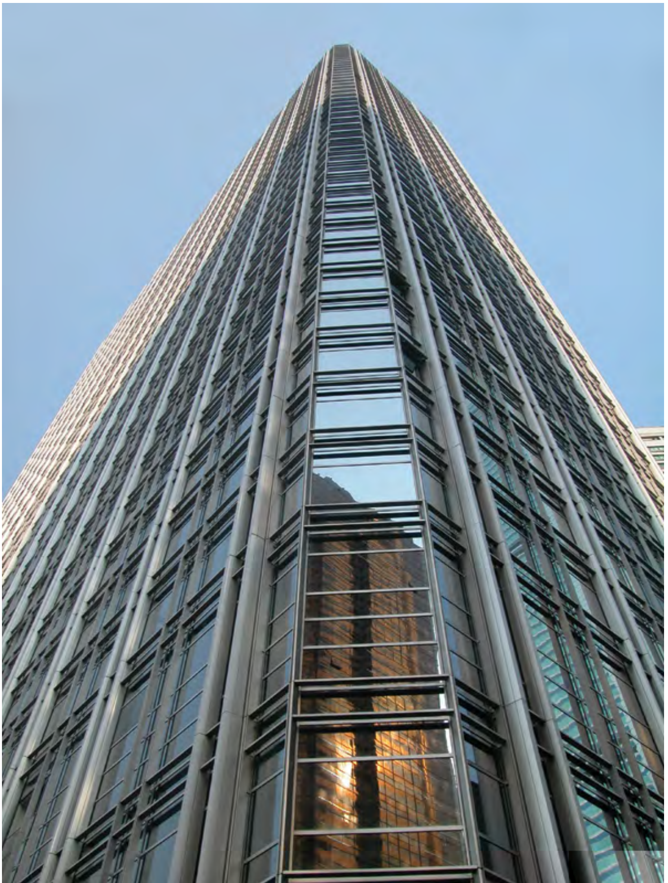
Unitized aluminium curtain wall system with Low-E glazing provides comfortable working environment and energy conservation
