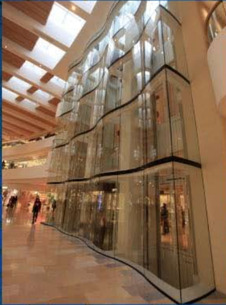
Curve Bubble Lift Enclosure, Pacific Place, Hong Kong
