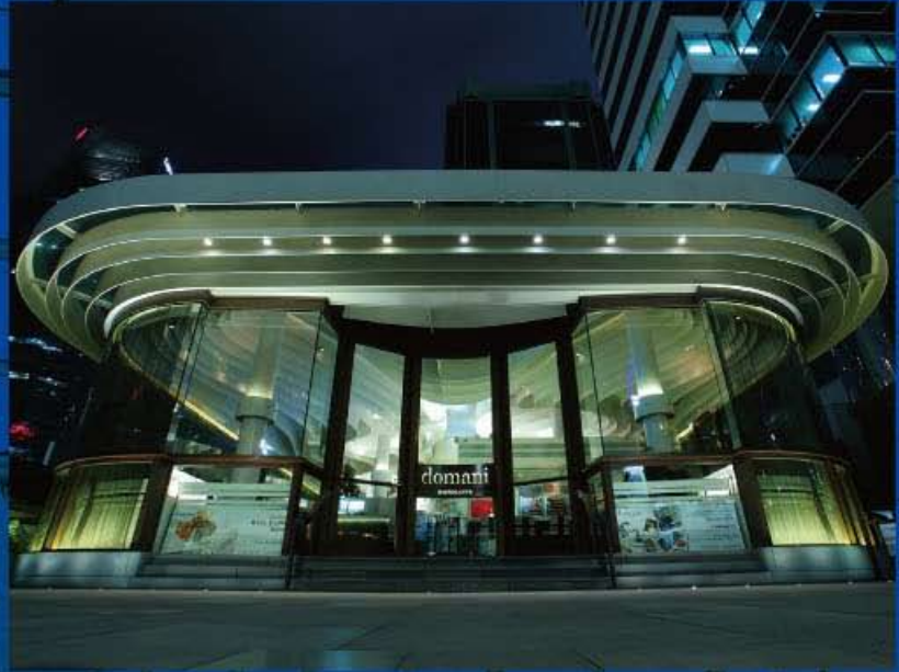
Canopy and Glass Enclosure, "Domani", Pacific Place, Hong Kong
