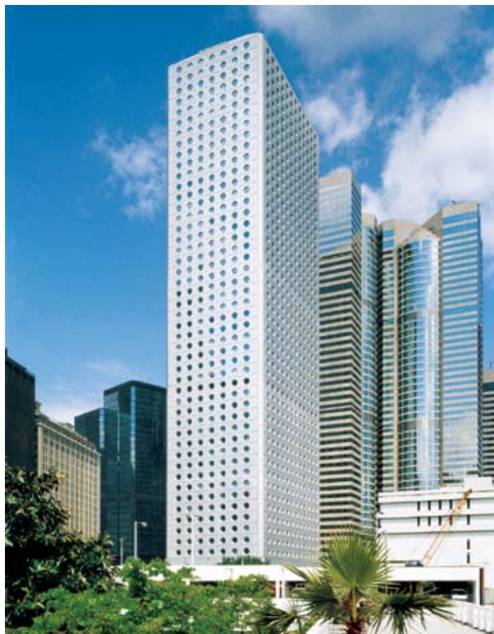
Connaught Centre (now known as Jardine House) : A Dow Corning project completed in 1973
