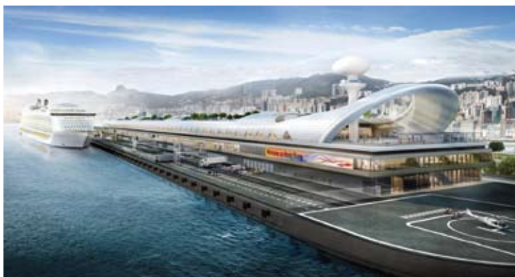
Kai Tak Cruise Terminal Building
