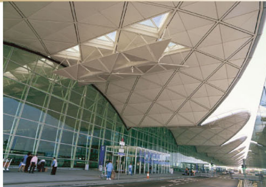
Hong Kong International Airport
