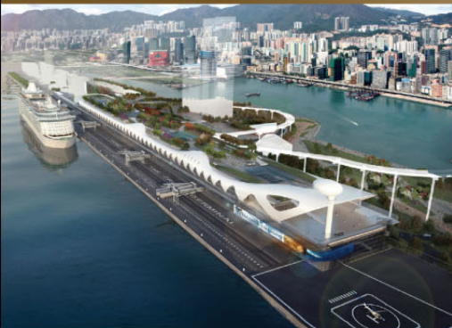
Kai Tak Cruise Terminal Building
