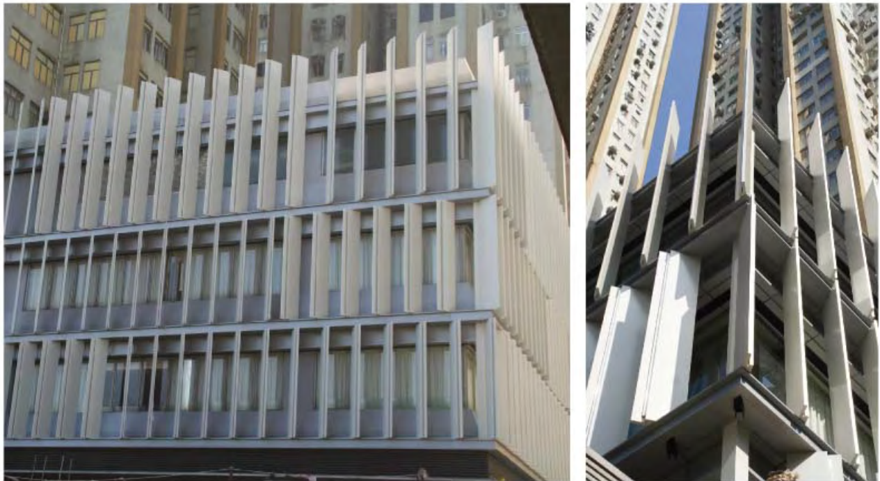
Renovation Work of Causeway Centre
