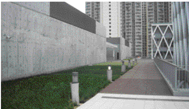
Use of fair-face concrete as external wall finishes for the plant rooms located at sky garden at 9/F of HKDI building
