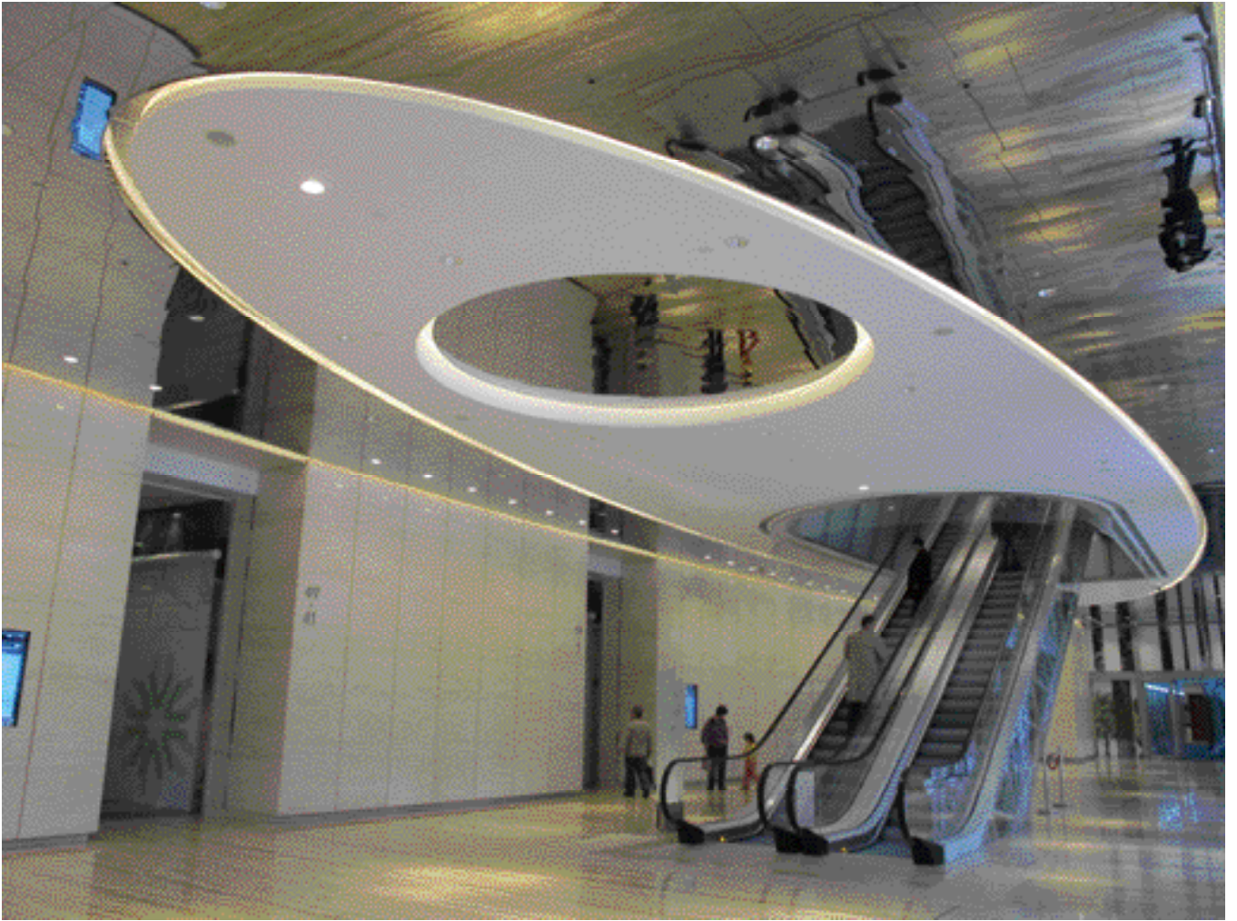
Renovation podium lobby at G/F
