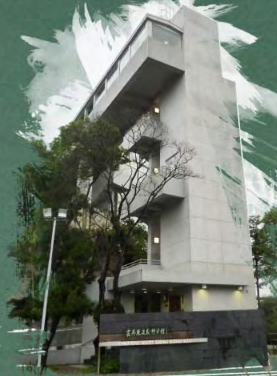
Fok Ying Tung Remote Sensing Science Building (The Chinese University of HK)
